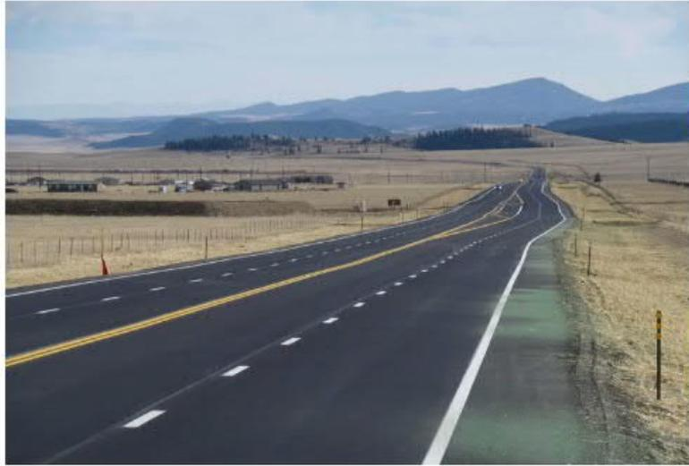
Figure 4-2 U.S. Highway 285 Passing Lanes. Photo credit: CDOT
